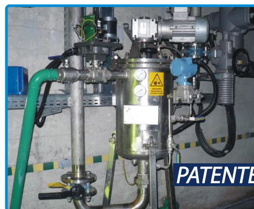
Self-cleaning filter for technological water DN 100 with manual drive
